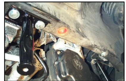
Figure 55 - Driver side frame rail ready to accept FMJ panel
