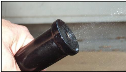
Figure 48 - Spray the female threaded hole of both of the front mounting posts with WD-40 or equivalent spray
